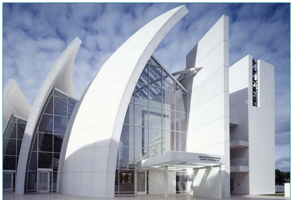
Figure 2: The “Jubilee Church” in Rome, built with photocatalytically active, “self-cleaning” concrete made by the company Italcementi. (Source: quartier-magazin.com/quartier08/der-weise-riese )
