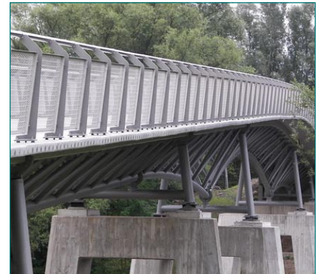
Figure 1: The Gärtnerplatzbrücke across the Fulda in Kassel River, made of ultra high performance concrete (Source: www.gaertnerplatzbruecke.de )
