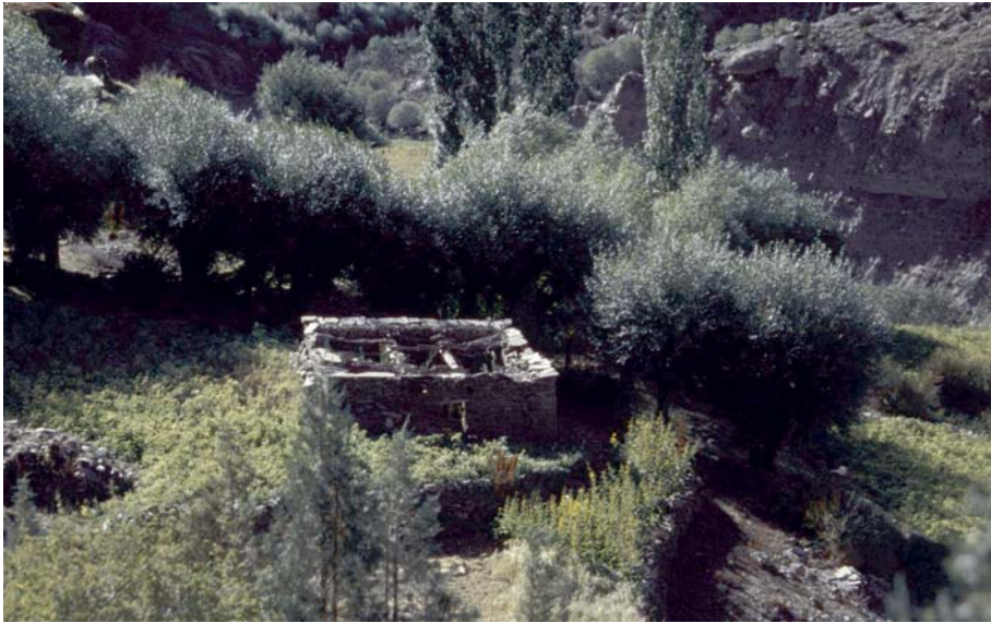
Figure 7.6 Collapsed temple of Johling. Photo: V. Widorn 1998.
