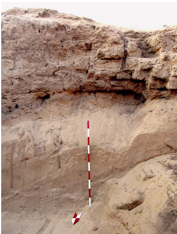
Fig. 4 Photo of the sand foundation under the Migdol gateway (L. Hudáková)
