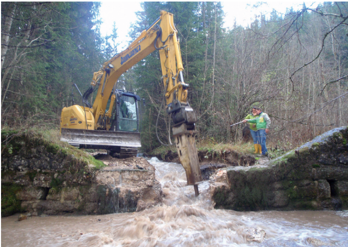
Figure 6 – Heavy machinery breaks through the barrier and the river bed becomes continuous again. © H. Haseke
