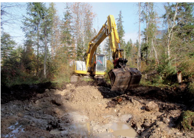
Figure 7 – Heavy machinery dredges a pond. © H. Haseke
