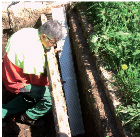
Figure 9 – Small metal ramps provide an exit route from the cattle grid. © H. Haseke
