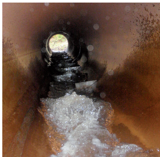
Figure 10 – Specially adapted pipes help the crayfish to pass under forest roads. © H. Haseke
