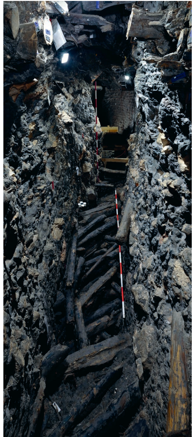
Fig. 5. Various views of fractured mine timbers at the Christian von Tuschwerk area (Photo: D. Brandner, NHM Vienna).
