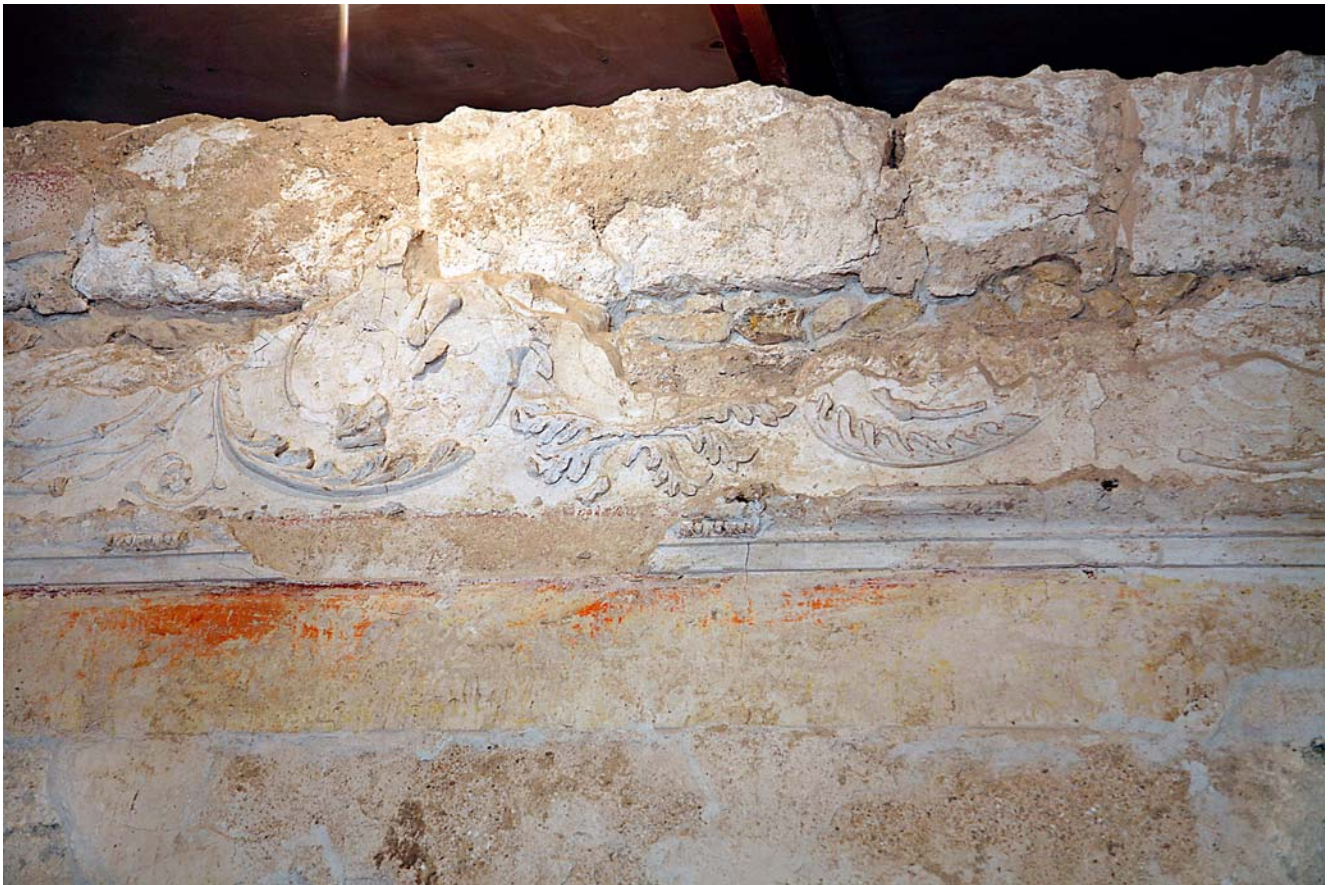
Abb. 10: Floral scroll in stucco of the entablature frieze at the top of the walls
