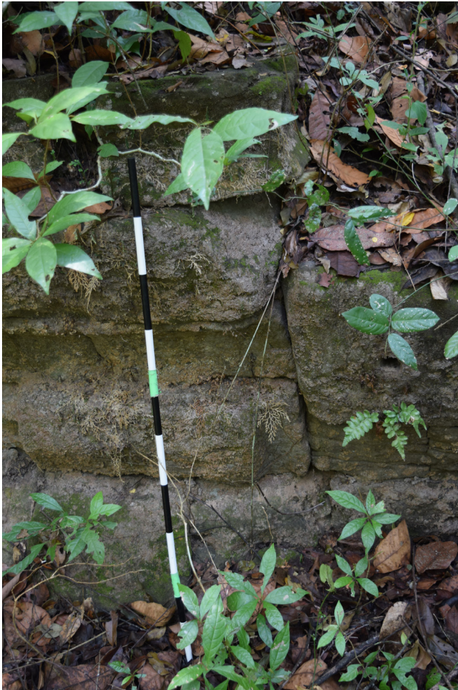
Fig. 6.0 (2): Architectural »break« between vihāra and original building, Terrasse Bouddhique No. 4 (ATV009). Shown referenced on original drawing of Buddhist terrace by Henri Marchal ( Monuments Secondaires, Pl. X )
