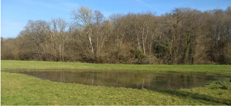
Figure 2: The primary scrape installed on reconnected floodplain adjacent to Cockhaise Brook in order to attenuate floodwaters.
