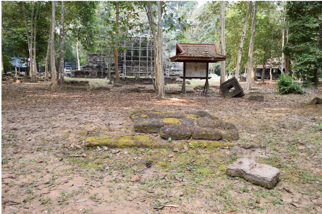
Fig. 1.0: Remains of laterite staircase to and from Western Prasat Top Temple and Buddhist terrace facing a cleared »local« road.
